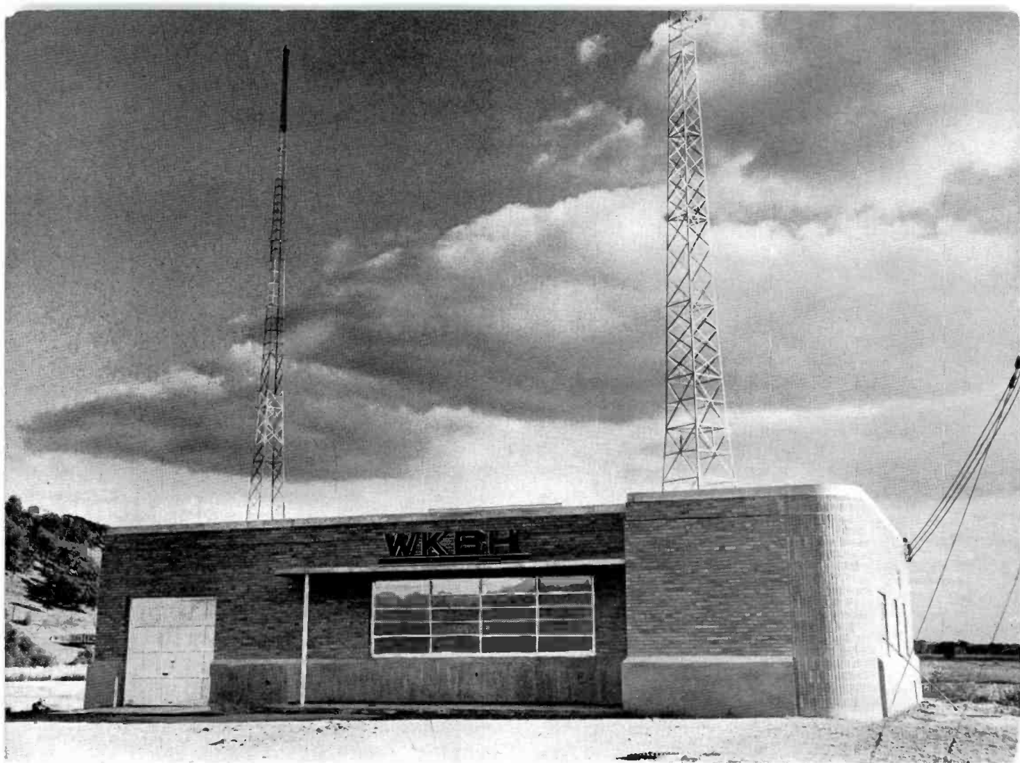
View of the New WKBH Transmitter Building with its Two-Element Directional Antenna Array.
