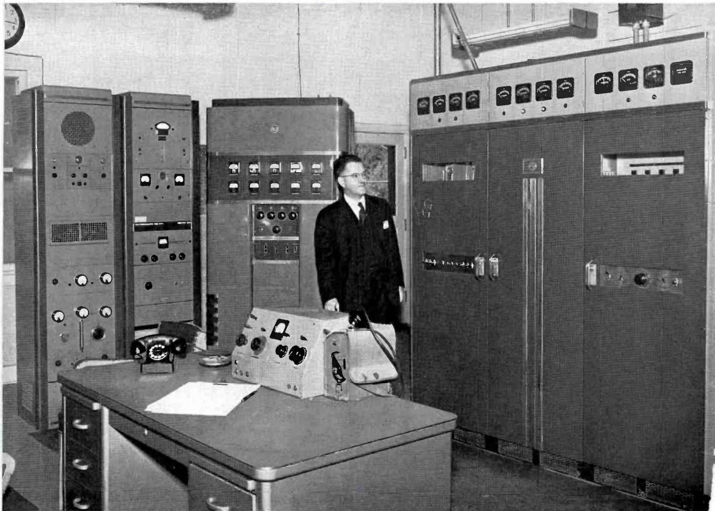
FIG. 1. Mr. Harold L. Dewing, President of WCVS and WCVS-FM has reason to be proud as he surveys his newly installed BTF-3B FM transmitter. Note how the well-planned transmitter room layout makes every piece of equipment convenient to the operator.
